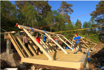
The main beams are raised during construction of Stakkslettua
