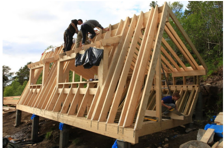
The rest of the cabins structure is built
